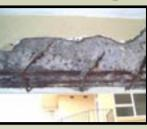
PRIOR REPAIR FAILED TO HALT IN-STEAD JUST HID THE CORROSION
