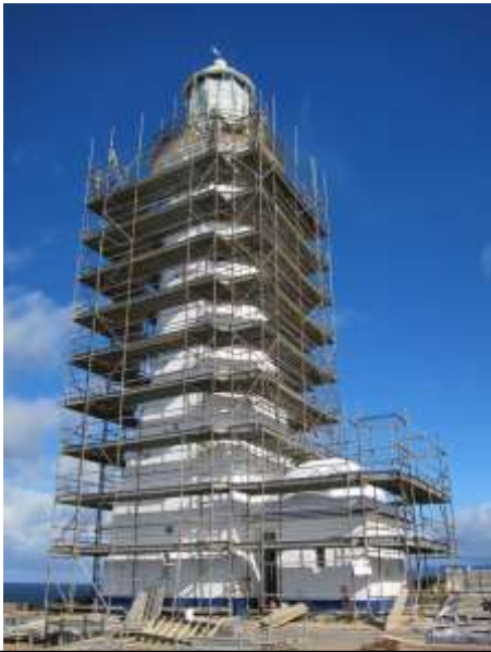
Scaffold being built encasing the Lighthouse structure.
