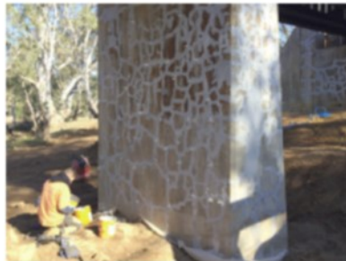
Concrete column being prepared for crack injection.
