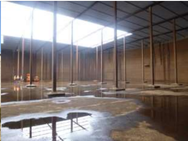
Figure 2 Internal view of a concrete tank with columns (roof partially removed)
