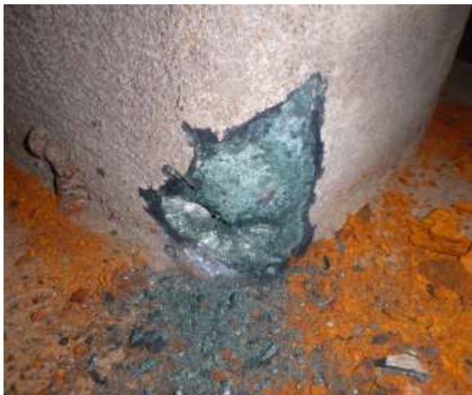
Figure 12 Concrete column surface after removing rust tubercles
