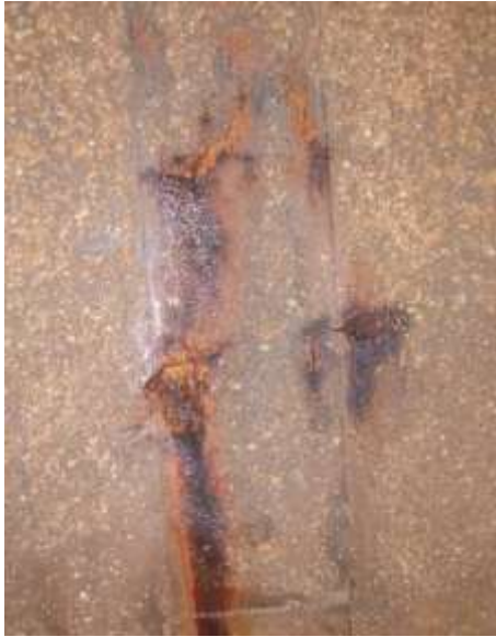
Figure 5 Visual appearance of concrete surface with evidence of steel reinforcement corrosion within the wall
