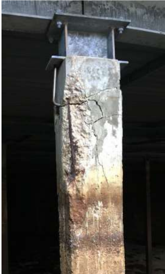
Figure 9 Top of column showing corroded reinforcement with low cover and concrete cracking
