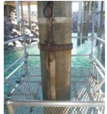
Photo: Work platform around concrete piles to complete crack and spalling repairs
