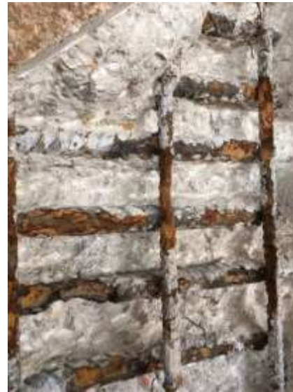
Figure 6 Reinforcement condition of the area identified in Figure 5 after concrete was broken away
