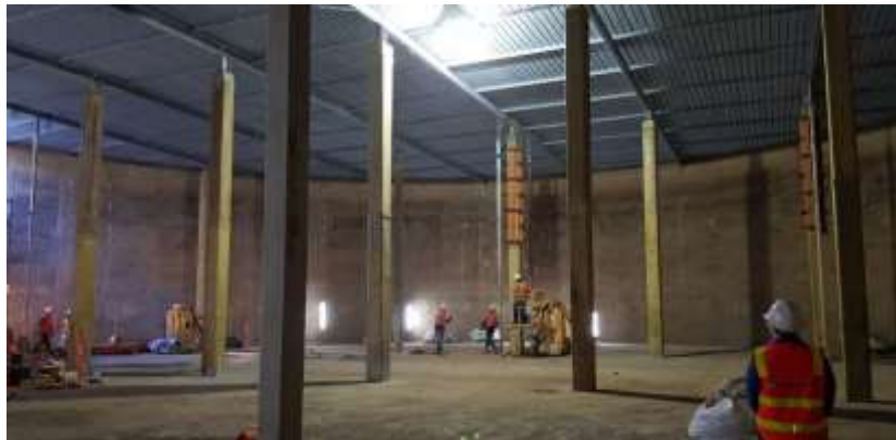
Figure 7 Columns rehabilitated with fibreglass jackets
