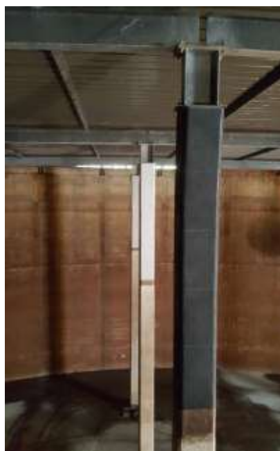
Figure 8 Columns rehabilitated with carbon fibre, columns at rear with an additional epoxy coating
