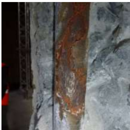
Figure 14 Pitted reinforcement
