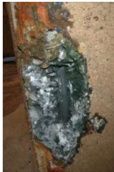
Figure 13 Exposed reinforcement at location where rust staining was evident on the column surface
