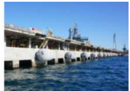
Photo: Work platform around concrete piles to complete crack and spalling repairs
