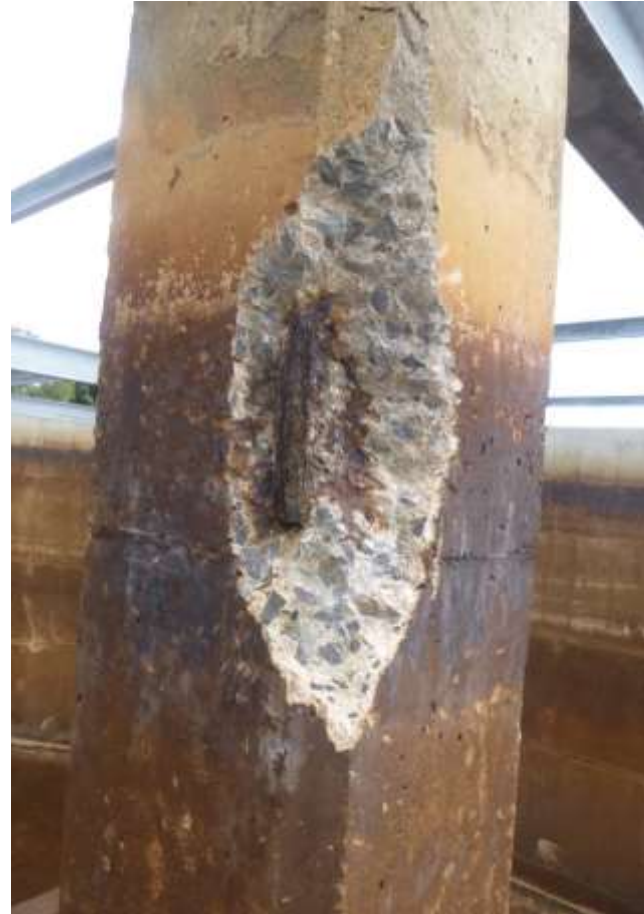
Figure 10 Top of column showing corroded reinforcement with low cover
