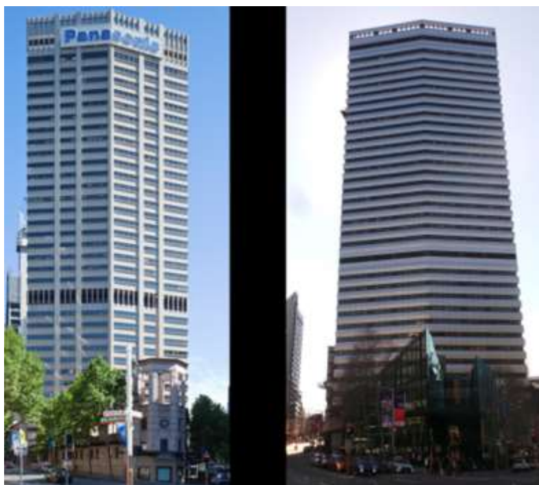
Northpoint, North Sydney - Before and After over cladding
