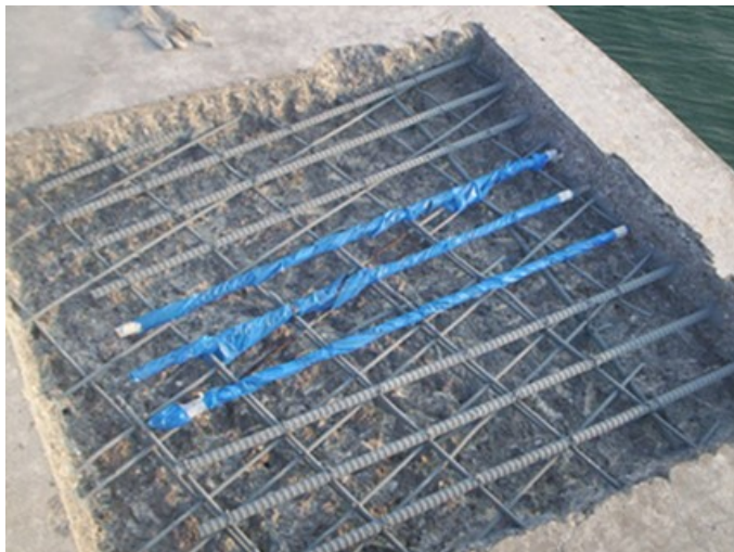
Figure 5: Steel cleaning and splicing by lapping after removal of concrete.
