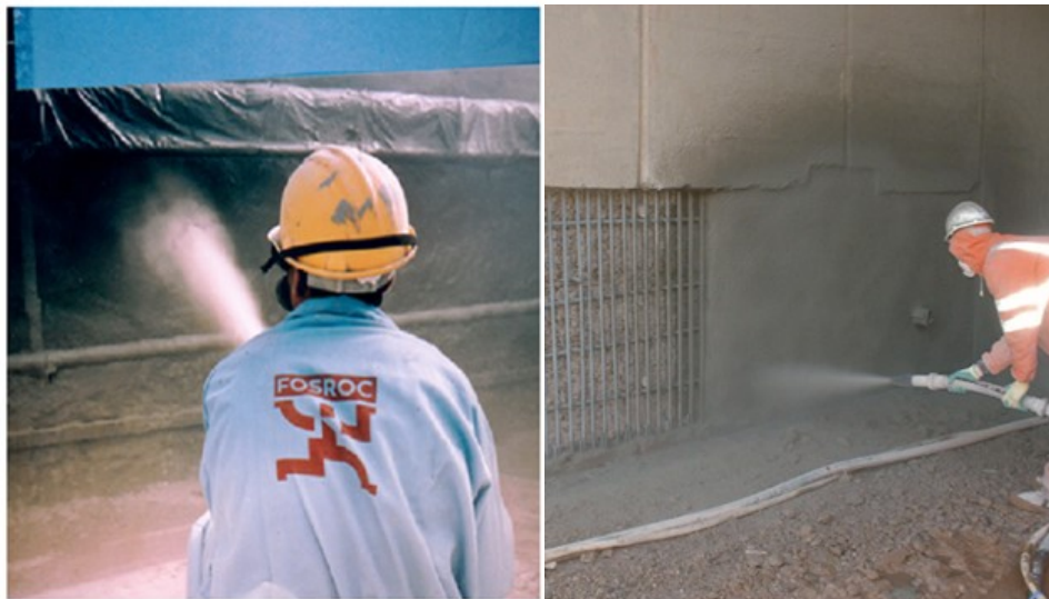
Figure 6: Sprayed repair mortars, in particular, do not require bonding agents as the shotcrete process exhibit excellent bonding characteristics by itself.
