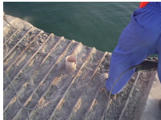
Figures 2 & 3: Impacting Method - Removal of deteriorated concrete by jack hammer.
