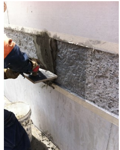
Figure 4: Concrete substrate is ready to receive repair materials after final surface cleaning.
