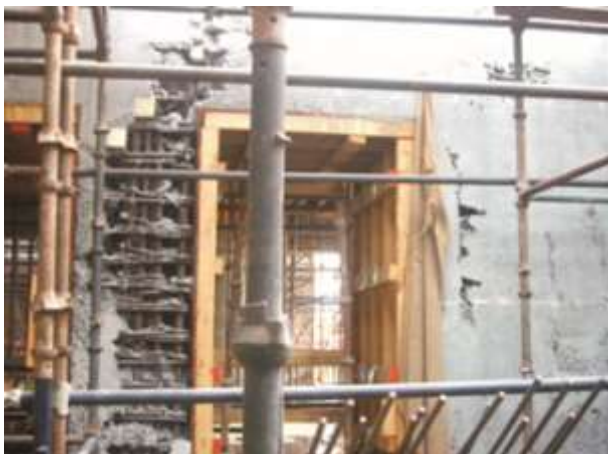
Figure 1: Honey combing defects in new construction
