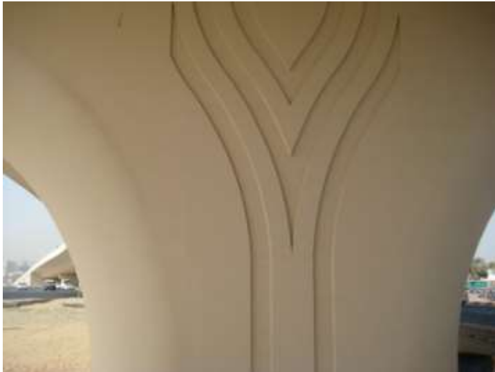
Figure 3: Bridge pier protected with anti-chloride and anti-carbonation protective coating after reinstatement with fluid micro-concrete mortar
