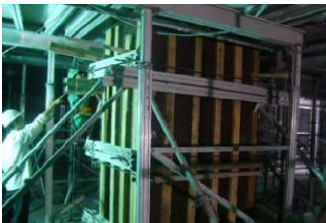
Figure 4: Form work in progress for fluid micro-concrete repair mortar as part of structural strengthening
