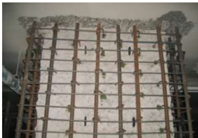
Figure 5: Structural strengthening of column using reinforced micro-concrete enlargement method
