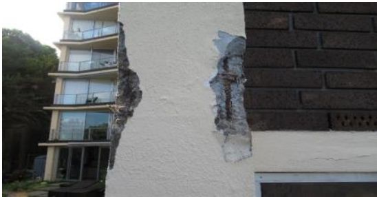
Defective repair and ongoing spalling
