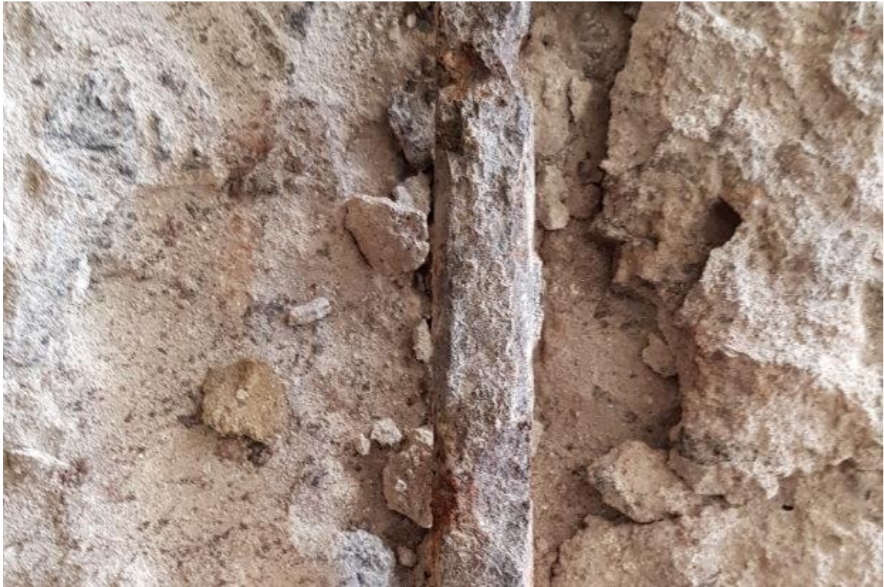
Signs of magnesite damage include cracked tiles and floors that bulge over rusting steel bars.
