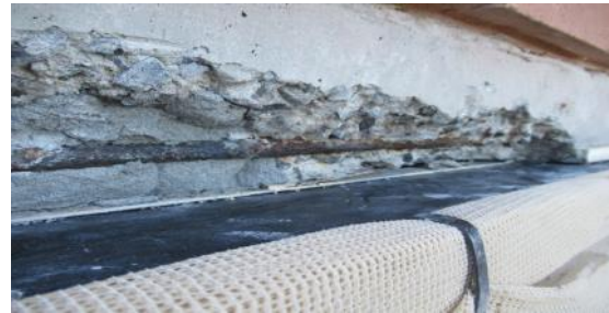
Slab degradation
