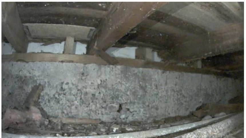
EQC failure: Attempts to "jack and pack" a ring foundation.
