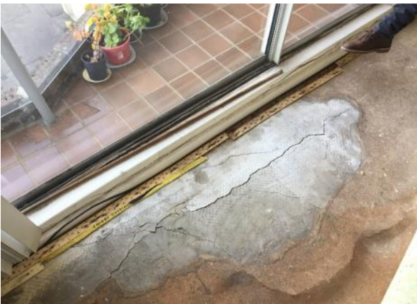
Magnesite floor that has not been properly remediated
