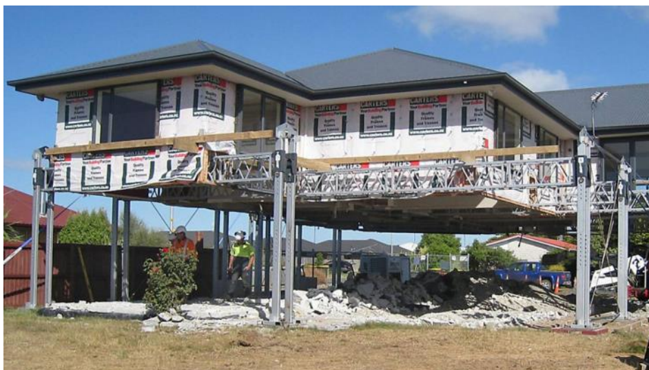
Doing it properly: How many houses should have been lifted and had their foundations rebuilt?
