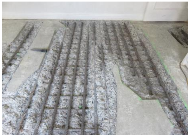
Magnesite floor remediation in action
