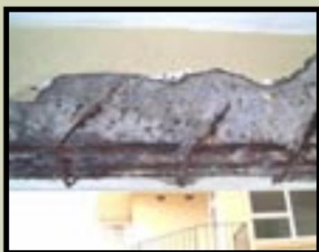
**PRIOR REPAIR FAILED TO HALT INSTEAD JUST HID THE CORROSION**
