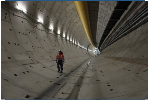
Photo: Waterview tunnel under construction © WSP
