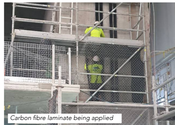
Carbon fibre strengthening
