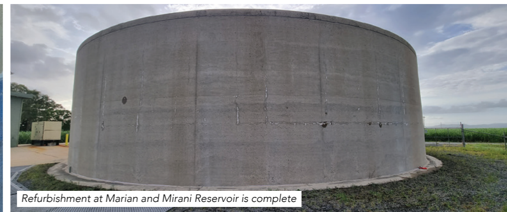
Refurbishment at Marian and Mirani Reservoir is complete
