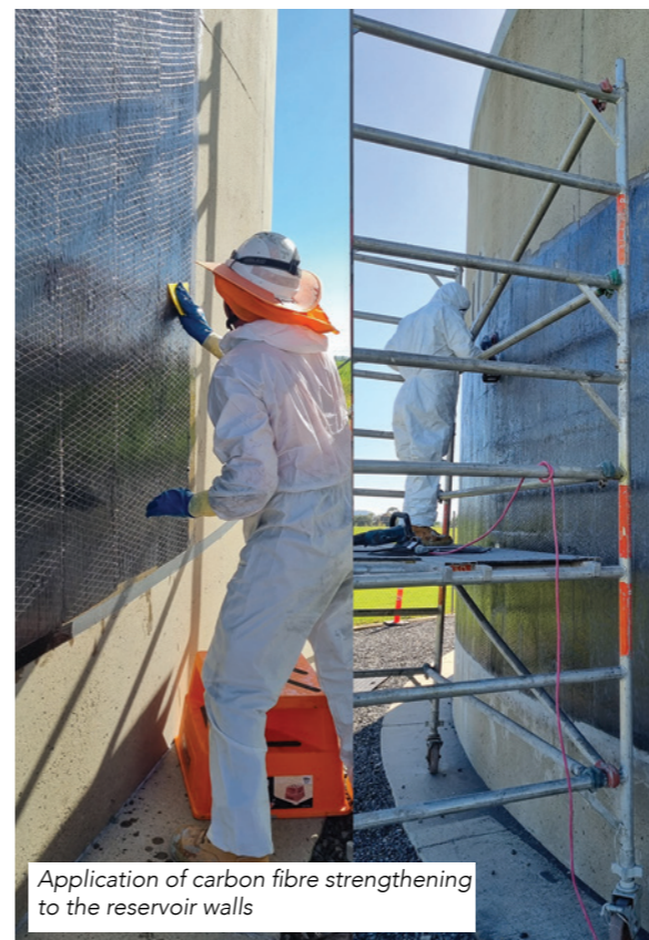
Repairing structural cracks
