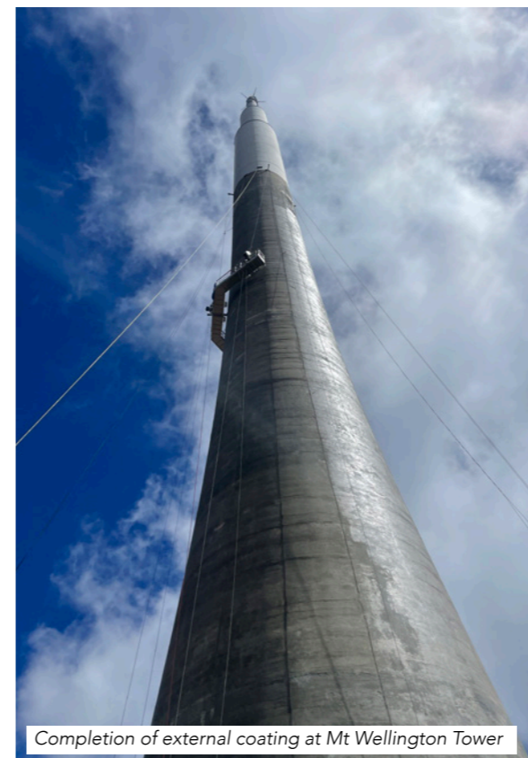
External coating at Mt Wellington Tower
