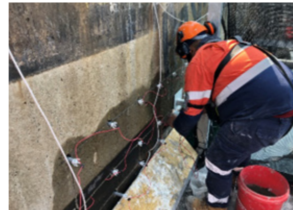
Installation of the cathodic protection system
