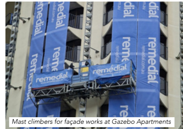
Containment sheeting installed on the balustrades to carry out the paint removal and reinstatement process.
