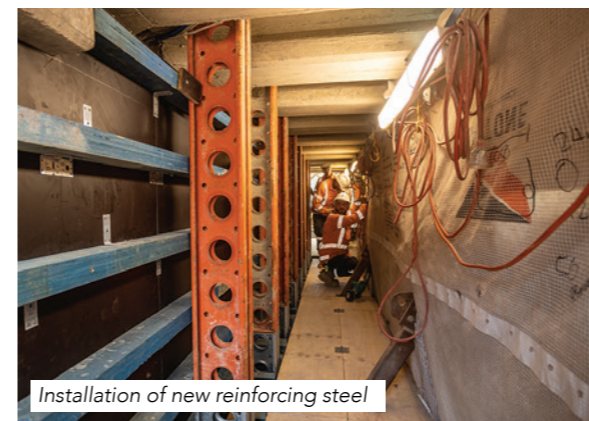
Installation of new reinforcing steel
