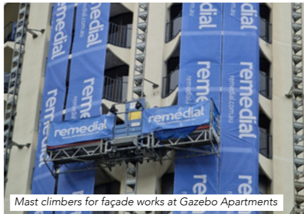
Containment sheeting installed on the balconies to carry out the paint removal and reinstatement process.
