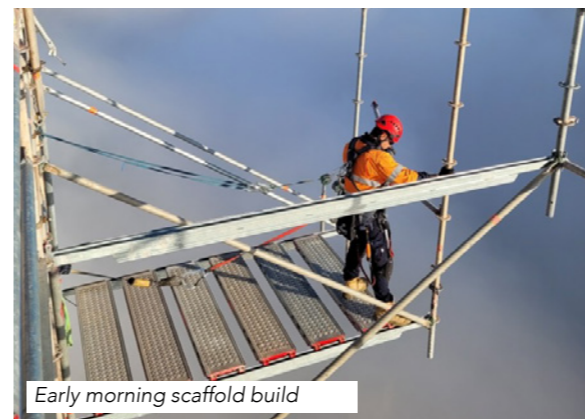
Rope access and netting
