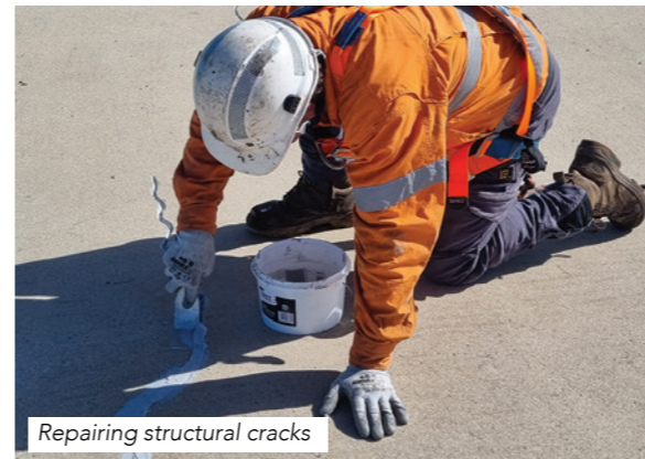
Repairing structural cracks
