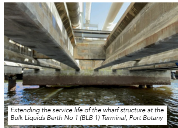
Underside of the berth
