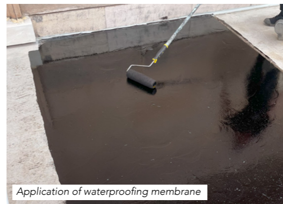
Balcony waterproofing works
