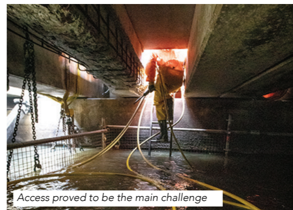
Concrete repairs at South Bank Parklands
