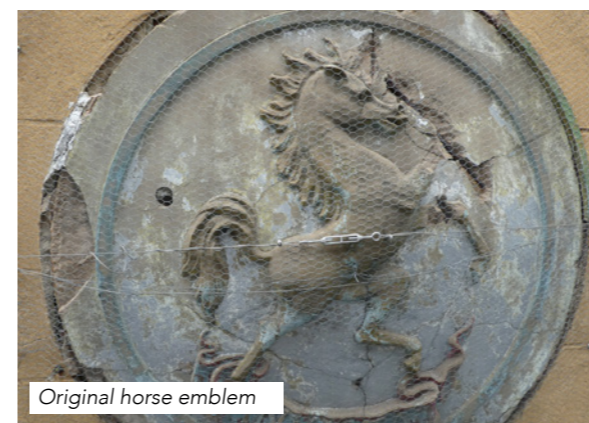
Façade restoration works
